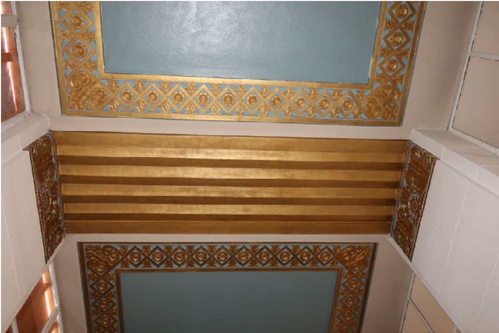
Fig.21 – Plaster ceilings
