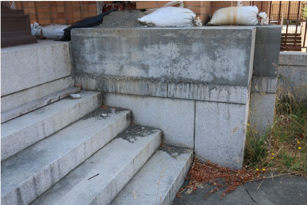
Fig.4 – Granite steps with added concrete abutment
