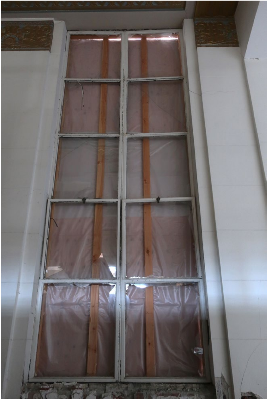
Fig.11 – Steel sash window (at interior)
