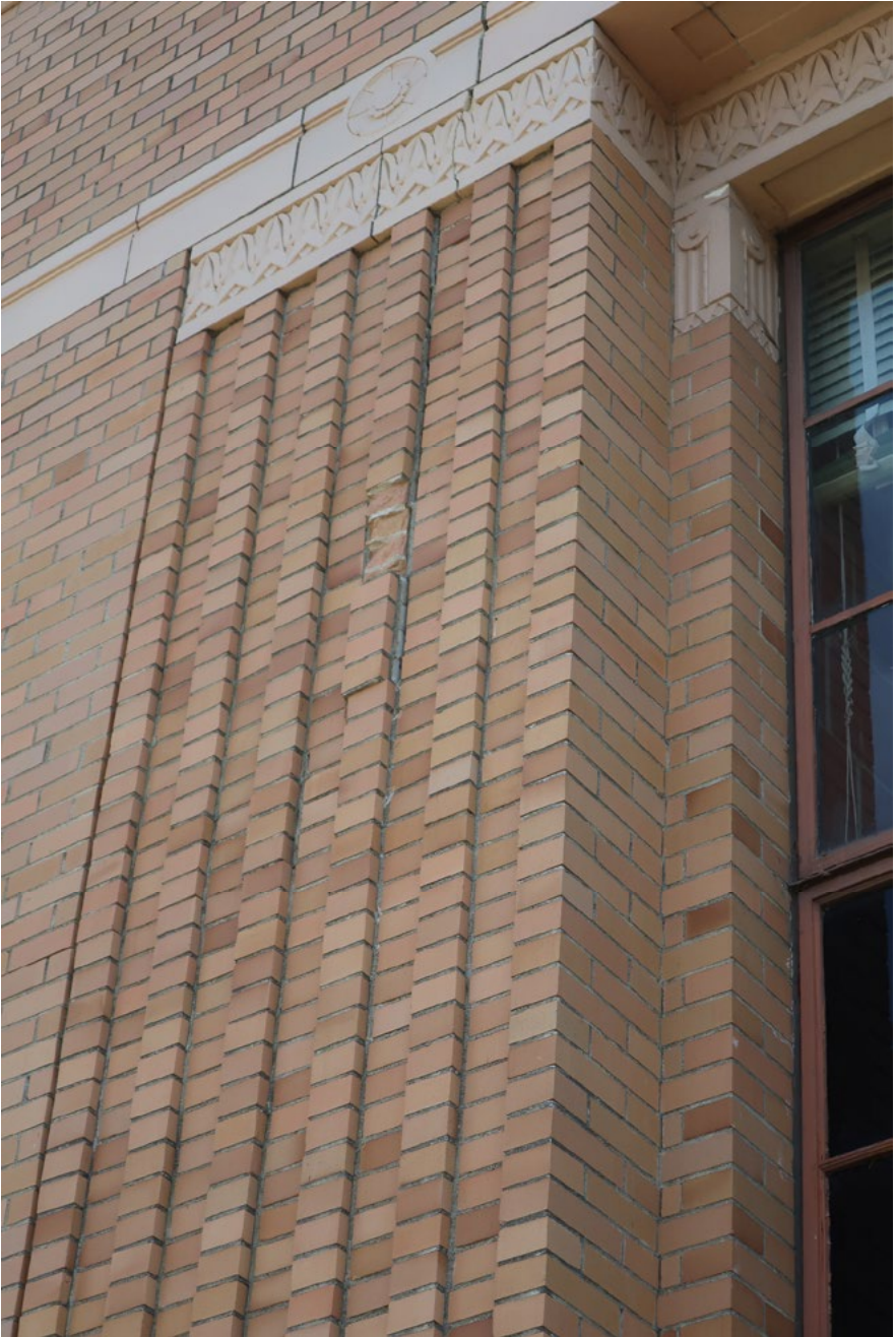
Fig.5 – Brick and terra cotta masonry
