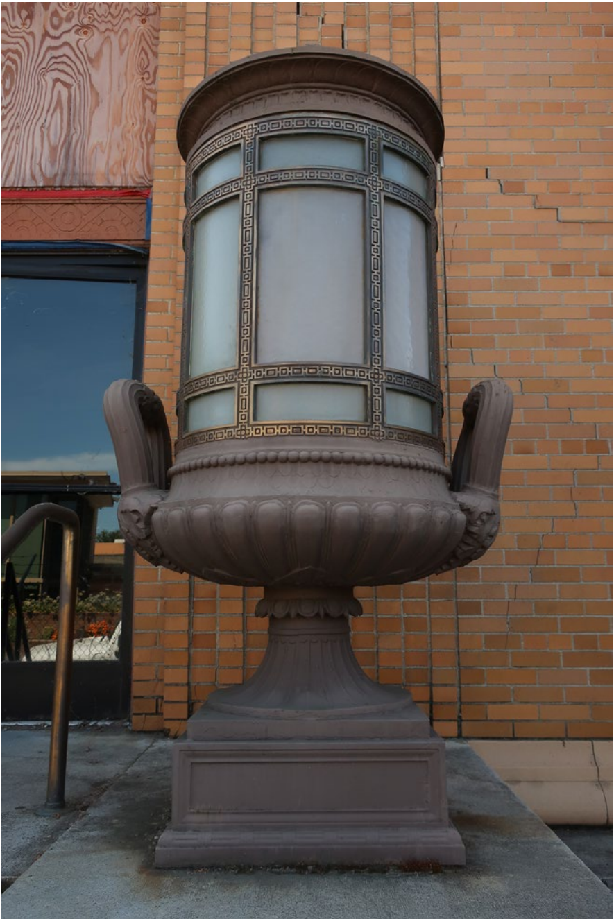
Fig.14 – Cast iron, bronze and glass lantern
