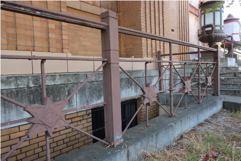
Fig.13 – Cast iron railing
