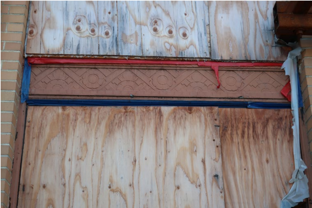
Fig.12 – Cast iron door lintel (and frame)
