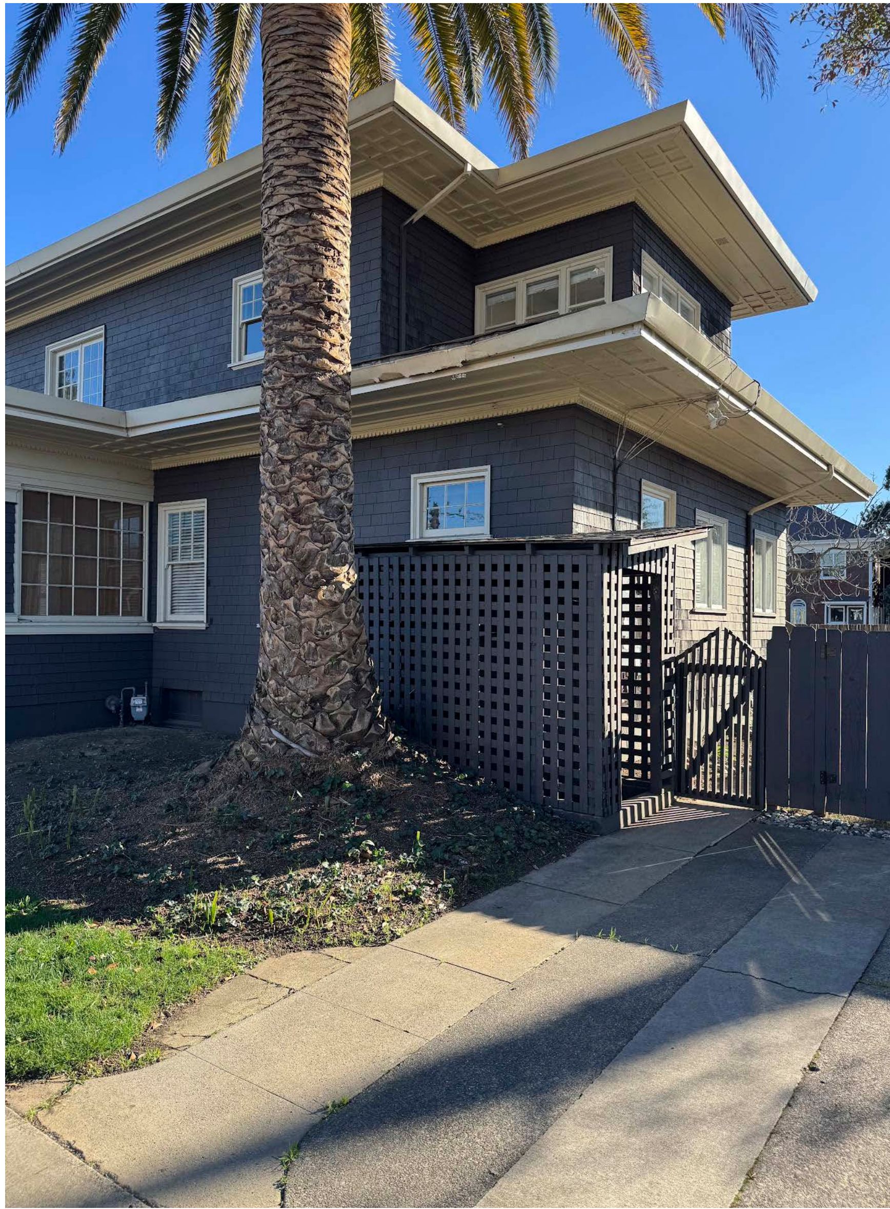
SECOND ST. NORTH-WEST CORNER VIEW
