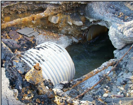
STORMDRAIN & CONVEYANCE REPAIRS
