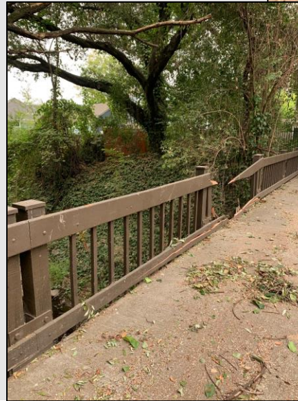
SENIOR CENTER BRIDGE RAILING REPAIR
