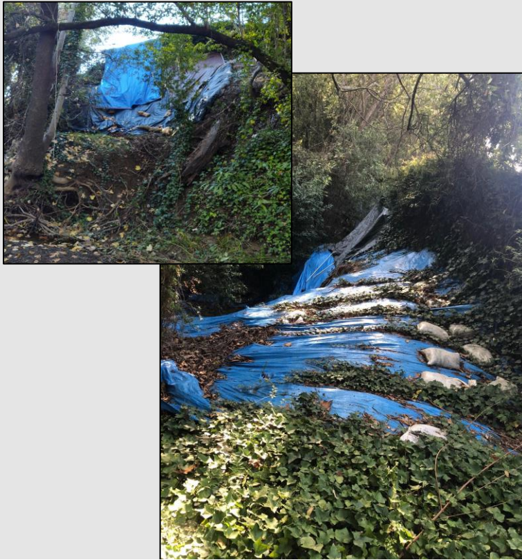
BROWNS VALLEY CREEK BANK REPAIR – BUHMAN PARK
