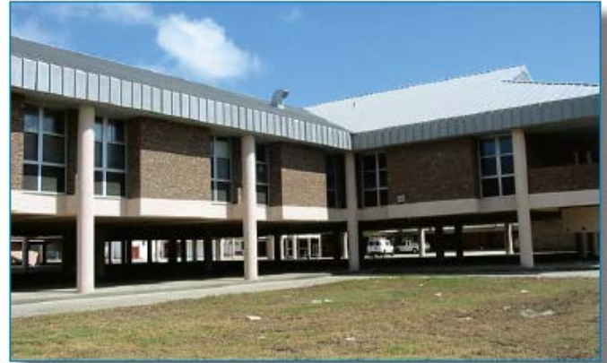
Figure 1: School elevated on columns
