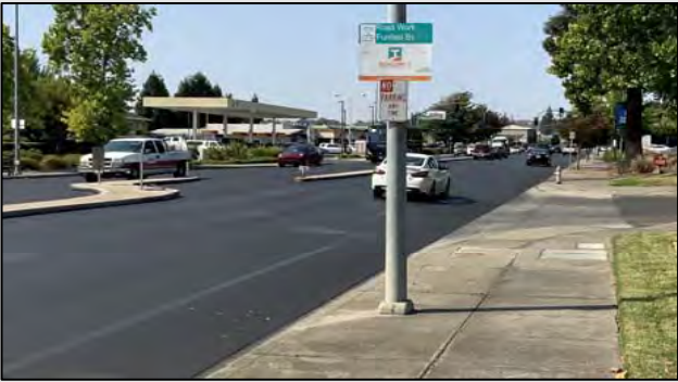
TRANCAS STREET REHAB
