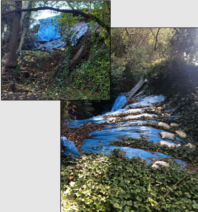
BROWNS VALLEY CREEK BANK REPAIR – BUHMAN PARK
