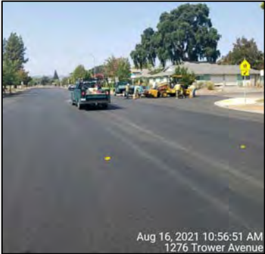
TROWER AVE REHAB PHASE 2
