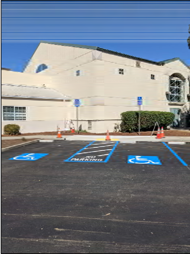
LAS FLORES COMMUNITY CENTER PARKING LOT REPAVING
