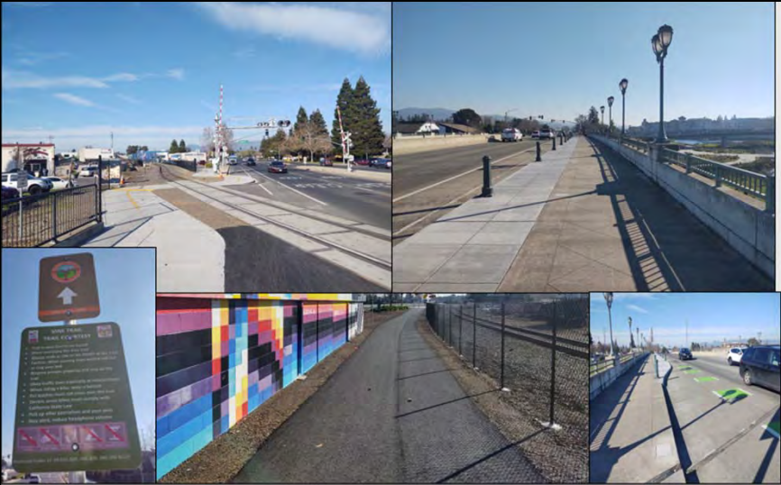
VINE TRAIL GAP CLOSURE* *INCLUDED FEDERAL GRANT
