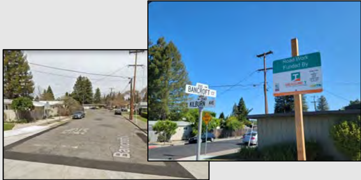
WESTWOOD REHAB PHASE 2A – BREMAN & BANCROFT COURTS
