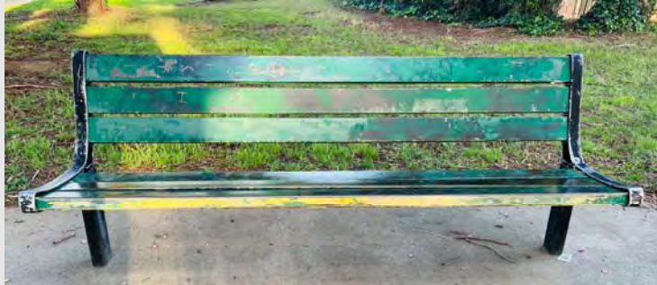
PARK AMENITY REPLACEMENTS
