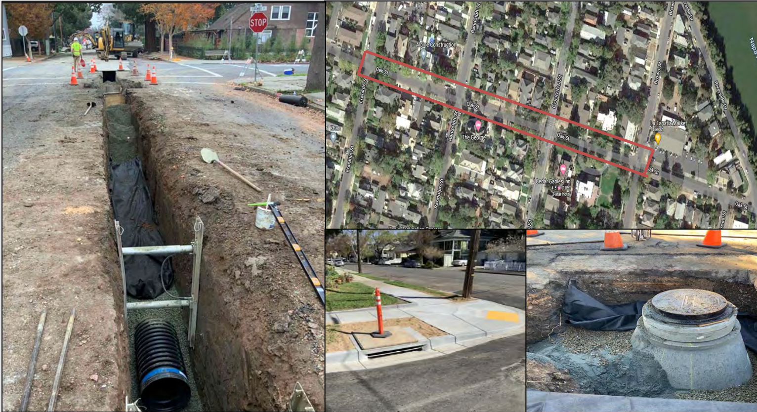
OAK STREET EMERGENCY REPAIR
