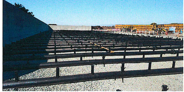
Under-Slab Air Pipes
