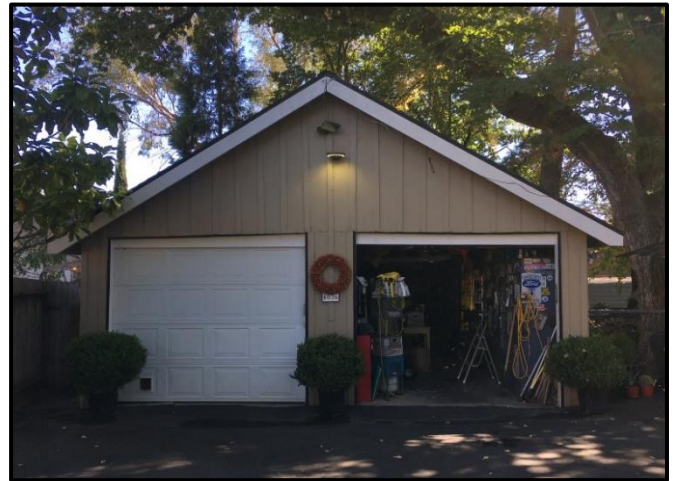
Image #45 – view looking east from Browns Valley road looking into rear driveway and parking area. Image #46 – view looking east to west elevation of historic carriage house. Note: The structure is covered with the original board and batten materials, the battens were hand hewn and not consistent dimensioned lumber. The only updates that have been done to the structure have been replacing the roofing materials, adding new garage doors on the west façade, and performing periodic painting of the exterior.
