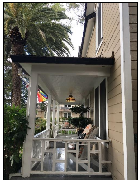
Image #31 – view looking south at original front porch. Original railing and beveled columns. Image #32 – original one over one double hung windows with ogee lugs. Original window trim.
