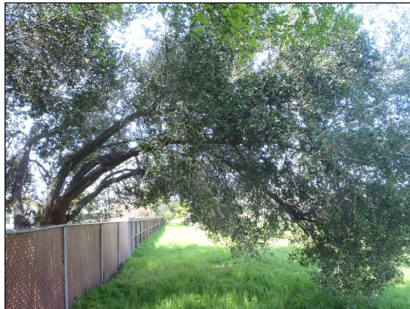
Photo 2: Looking northwest along the existing fence at the crown of coast live oak #326. I estimated that 90% of the crown extended approximately 23' east over fence and onto the development site. Pruning cannot correct this situation.
