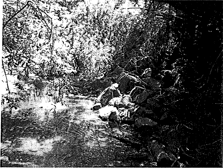
Photo 7: Downstream view along 40-50 ft. riprap treatment of the west bank adjoining the vacant Project building's rear parking area. Note the boulders encroaching on the active flow zone of the channel.
