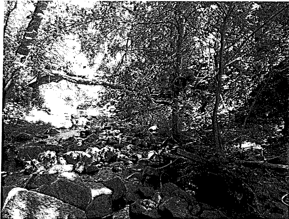
Photo 3: Downstream view along the roughly longitudinal and discontinuous mid-channel bar formed by collapsed boulders transported a short distance downstream from the upstream riprap revetments.
