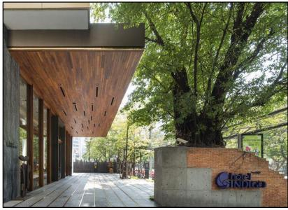
The shape, size, color, and material of projections for shade protection should be consistent with the architectural style/character of the building. The minimum dimensions of awnings should be consistent with the width of the glazing.
