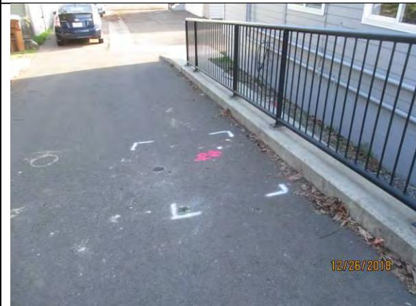
Backfilled probes and boreholes at SG-3/SB-3.
