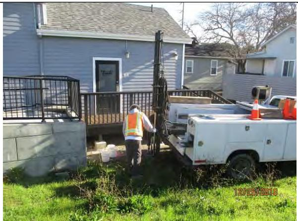
Drilling rig set up on sample location SG-6/SB-6.
