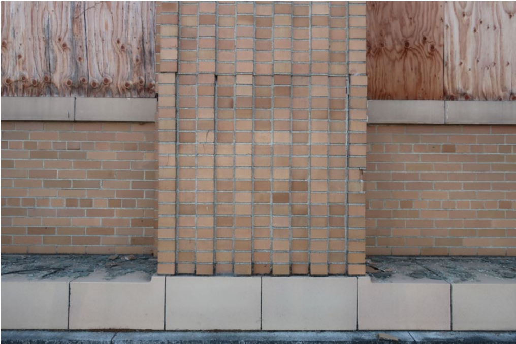
Fig.9 – Brick and terra cotta masonry
