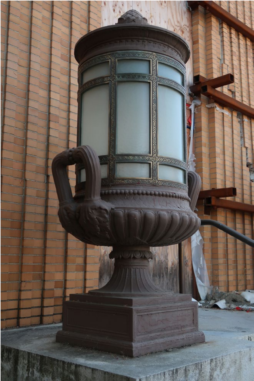
Fig.15 – Cast iron, bronze and glass lantern
