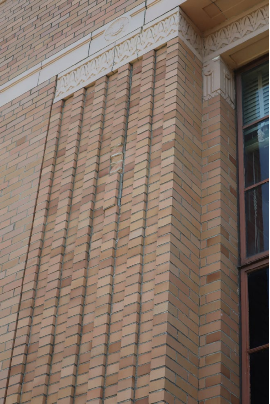
Fig.5 – Brick and terra cotta masonry
