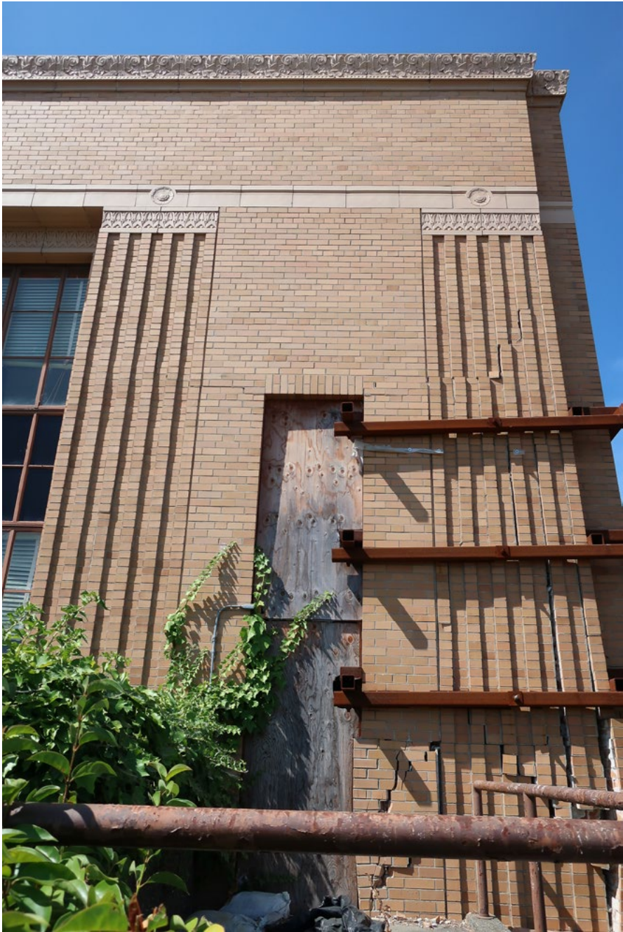
Fig.7 – Brick and terra cotta masonry
