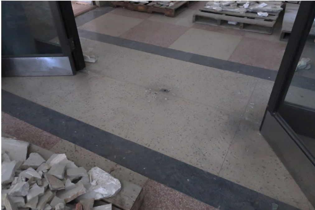
Fig.16 – Terrazzo flooring (with marble borders and bands)
