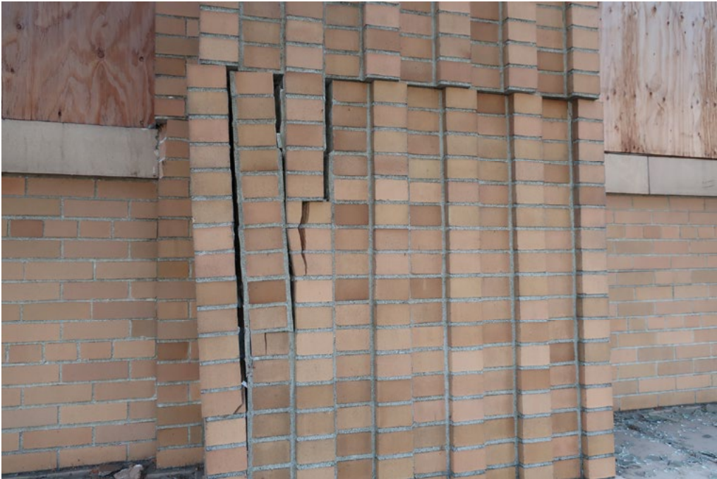
Fig.8 – Brick and terra cotta masonry
