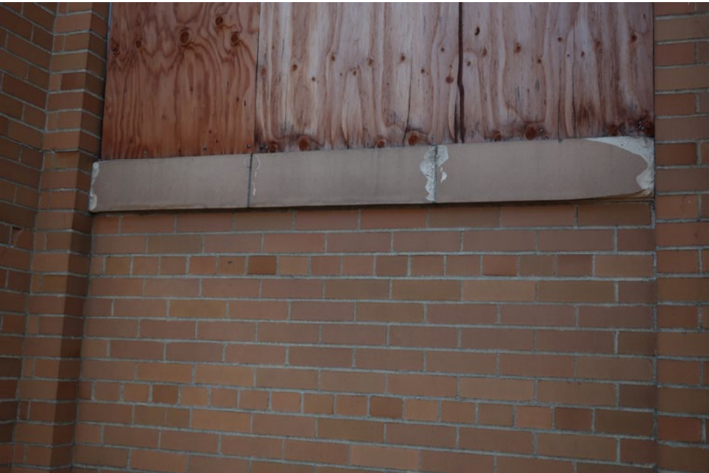
Fig.10 – Brick and terra cotta masonry
