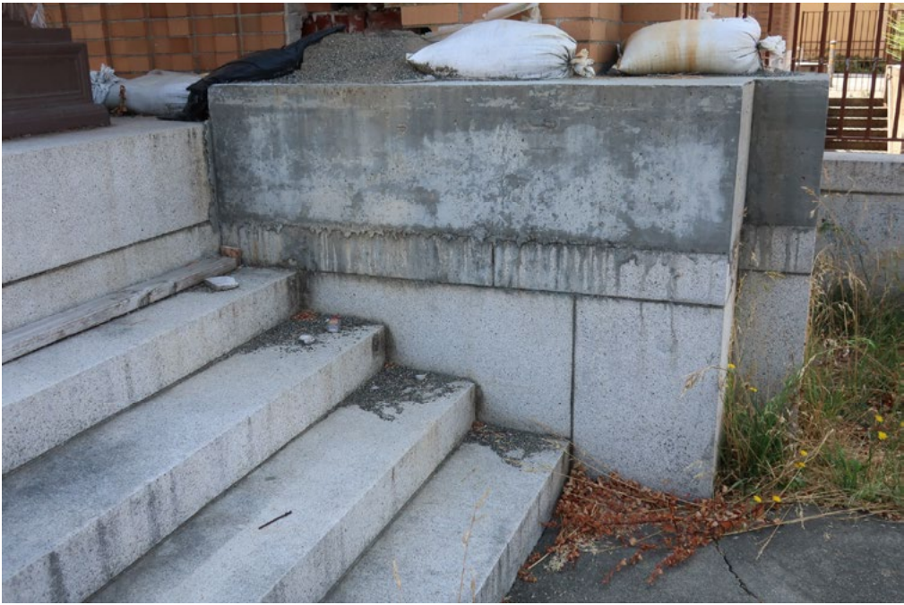
Fig.4 – Granite steps with added concrete abutment
