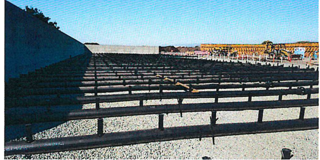
Under-Slab Air Pipes
