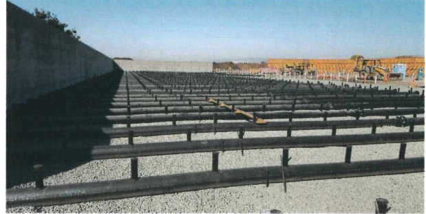
Under-Slab Air Pipes
