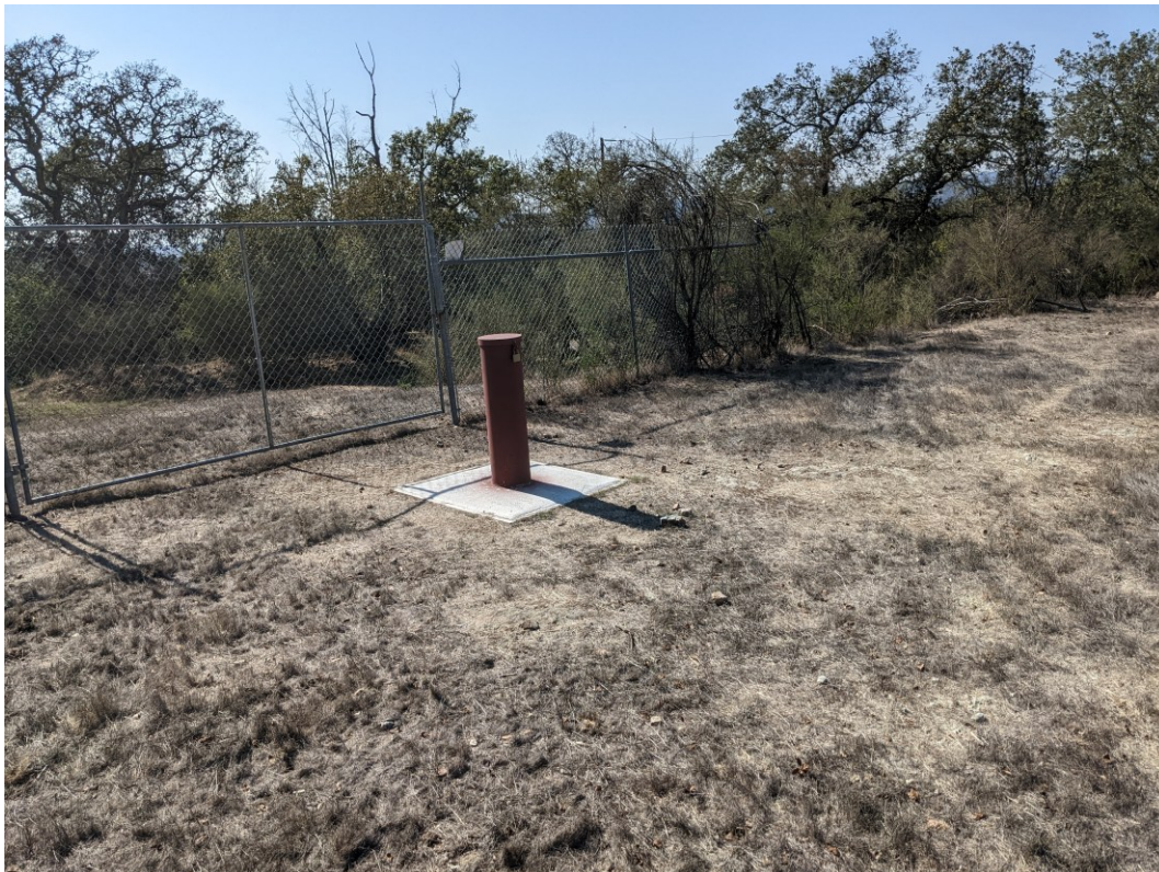
Photo 9 – Methane Gas Monitoring Well #2 Along Fence with Lot 7 (looking south-west)
