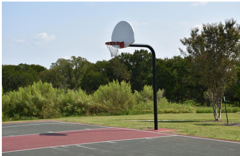
Pathway & Sports Court Rehabilitation
