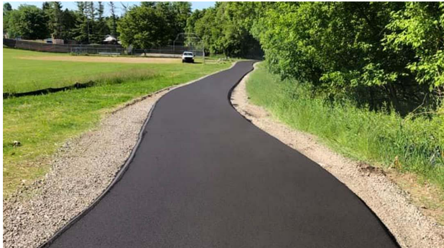
Pathway & Sports Court Rehabilitation
