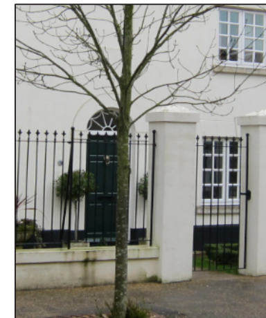
Stucco, finish, Windows
