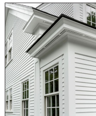
Soffit, Moulding, Trim, window
