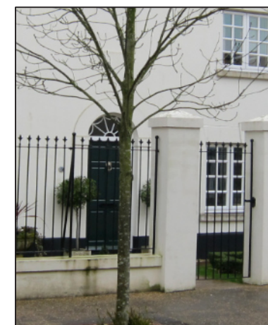
Stucco, finish, Windows
