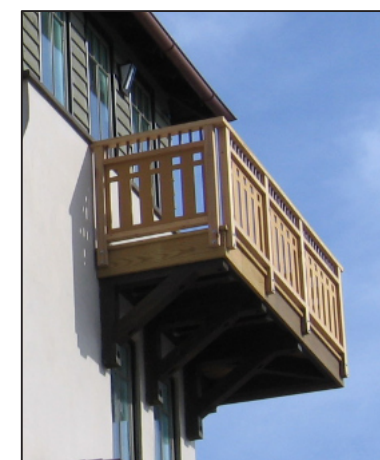
Wood finish, brackets
