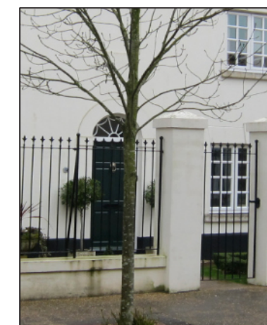
Stucco, finish, windows
