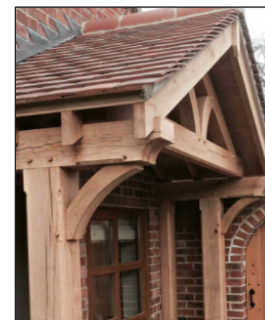
Brackets, Carpentry
