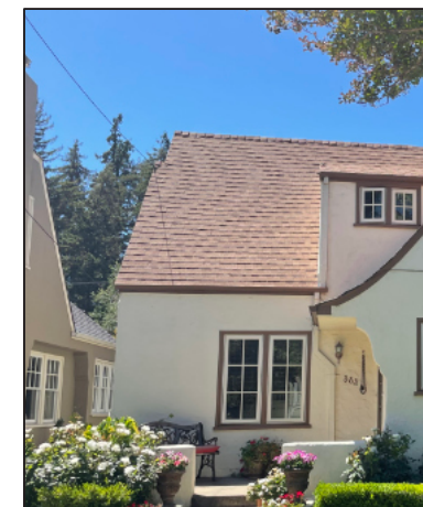
Shingle style / Stucco finish Window
