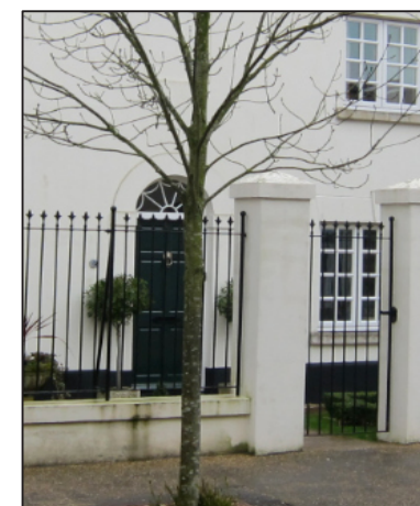
Stucco finish, Windows
