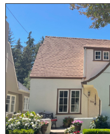
Shingle style / Stucco finish Window
