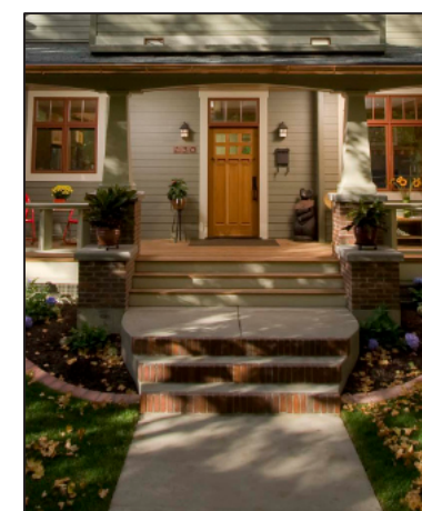
Siding, concrete, brick work
