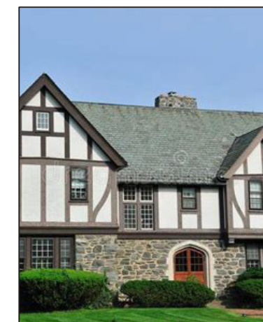
Timber details, windows
