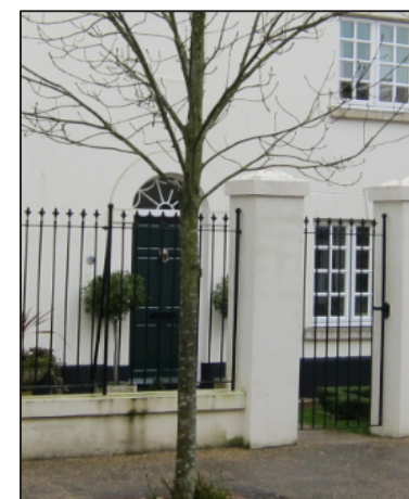
Stucco, finish, Windows
