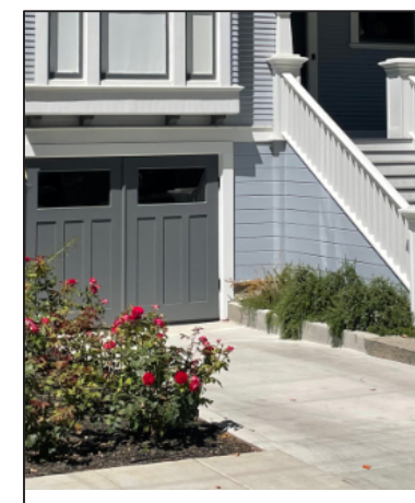
Rustication on foundation
