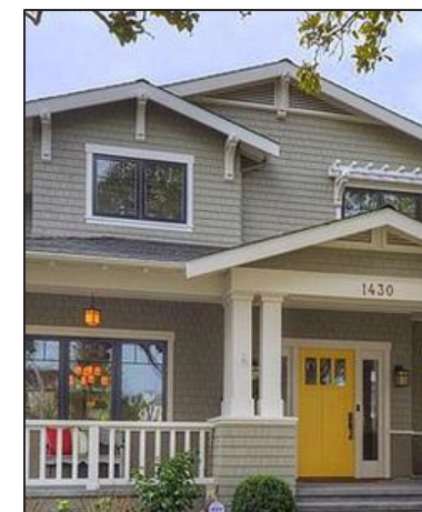
Siding, windows, trim
